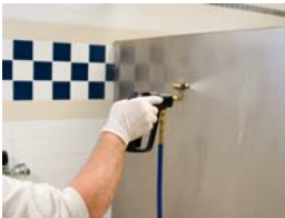
4. Spray walls and partitions
